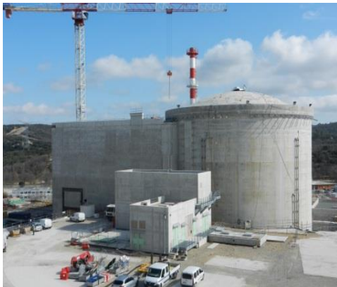
JHR Building site- Mid 2017
